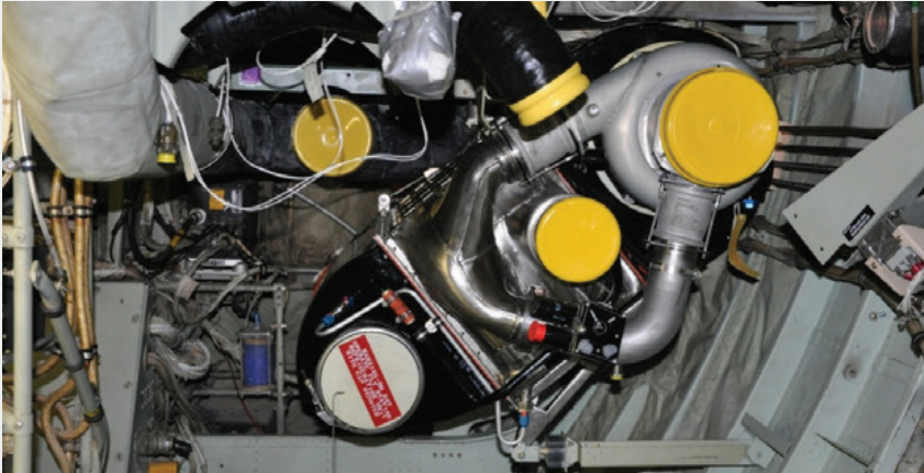
NEW ECS REFRIGERATION UNIT
