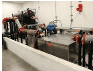
Fuel Flow Test
